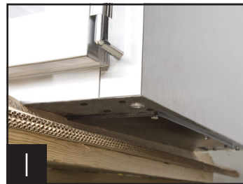
Slide packing material under the unit.
