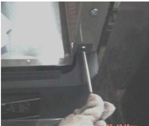
C. Unscrew screws on top grille (B).
